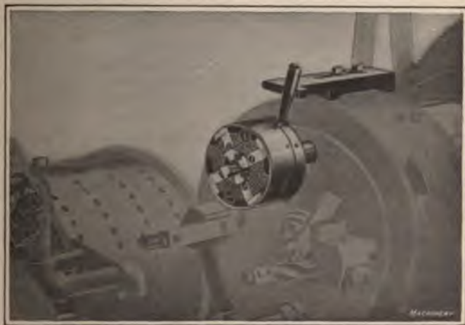
Fig. 9. "Namco" Self-opening Die-head on a Cleveland Automatic, showing Closing Device
